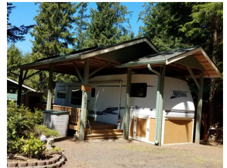
Figure 2: RV Roof Example
